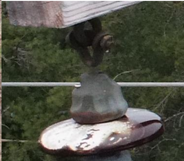
Figures 23 and 24: Component 3: Claytor – Fieldale 138-kV Line Structure 30-218: Moderate Vertical Pole Splitting and Flashover/Arcing Damage to Insulator
